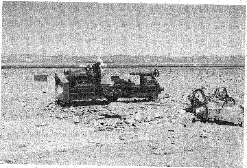
Figure 4.76a. Machine tools after the nuclear explosion (10 psi overpressure).
